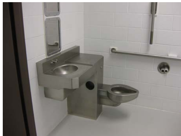
Isle of Wight Court Floor Holding Cell
